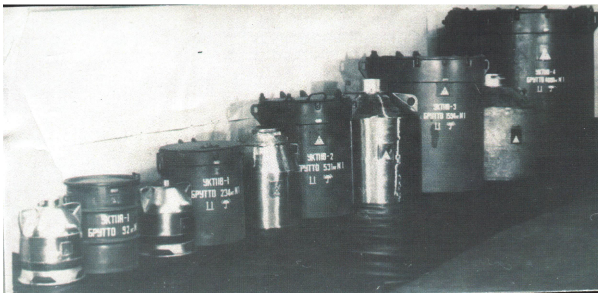
Fig.4: The unified line of containers for transportation of neutron sources
