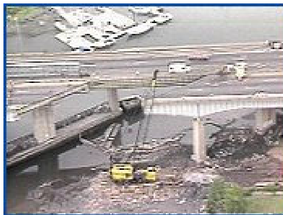
Figure 1: Cleanup of the collapsed span of the Mianus River Bridge
